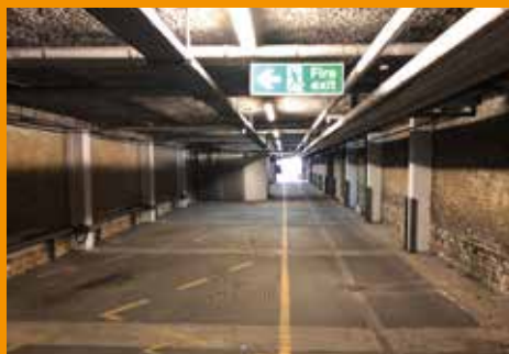
Existing internal view
