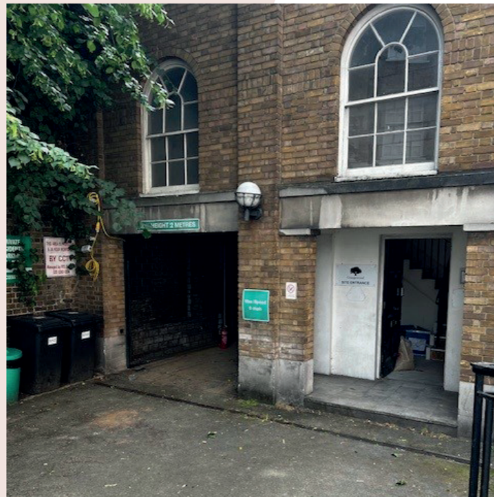
Existing entrance at 40 Pelham Street
