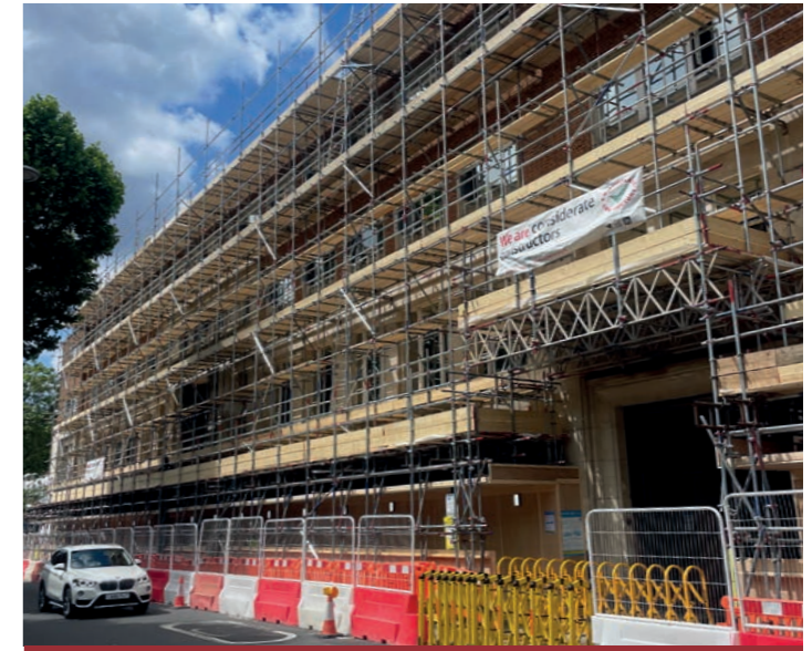
Setting up the scaffolding at 80 Pelham Street
