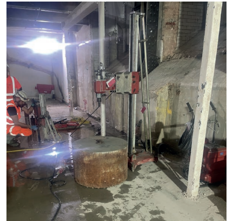
Stripping out the building at 80 Pelham Street
