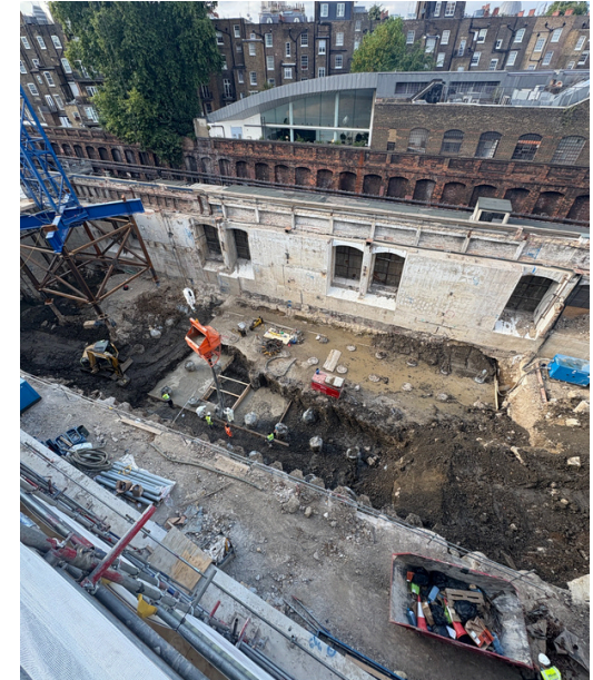
The new basement slab is about to be poured
